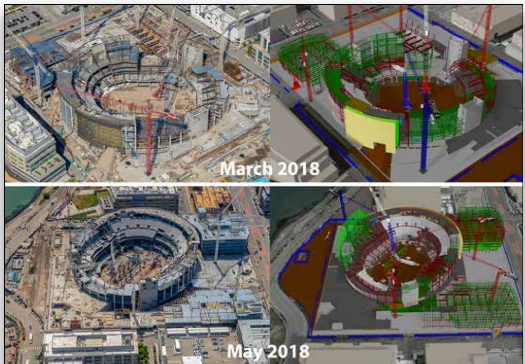
Using SYNCHRO for 4D visualization, Mortenson | Clark created 1,674 critical schedule activities with over 151,635 individual resource elements.
